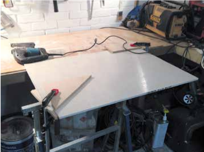
Securely clamp the solid surface material down, protecting it with offcuts of softwood, and carefully start cutting with your new jigsaw bit
